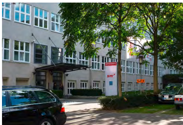
Bürocampus Wangen, Stuttgart-Wangen
